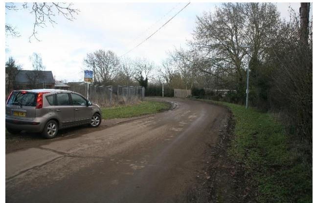
These photographs show the state of the road between the factory and the hamlet. It shows the state of the road, its width, its edges and potholes. It is seriously in need of repair and resurfacing.
