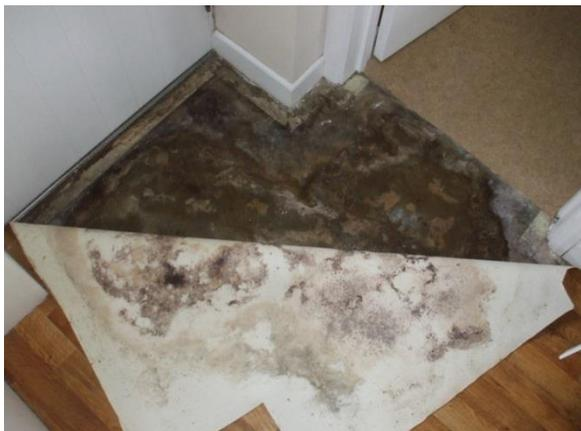
**Photograph 5:** Damp and mould hazard
